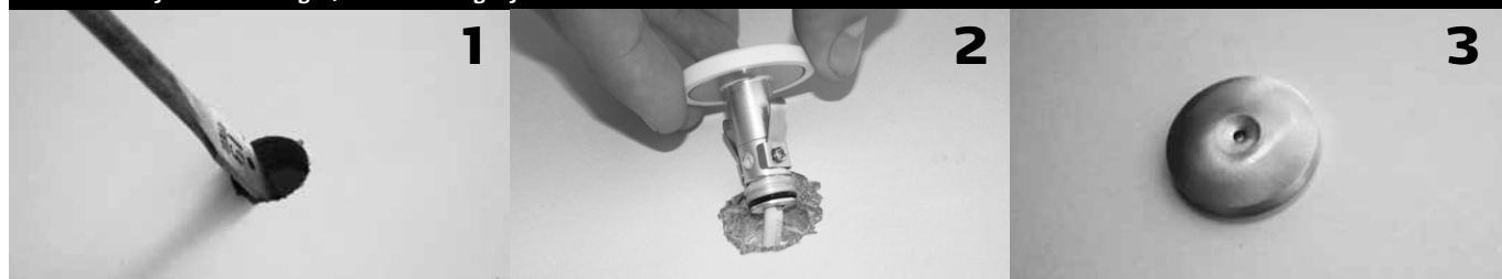
Installation of Mini Downlight, without using a flex tube.
